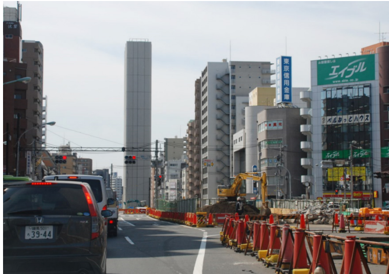
Figure 15: Yamate tunnel air exchange stacks (45 m high) at Yamate Street, Tokyo
