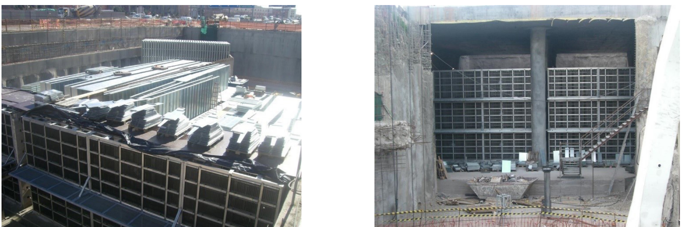
Figure 8: Left: Ventilation station PV4, ESP at the front, DeNOx plant at back. Right: Ventilation station PV3, ESP front view 25
