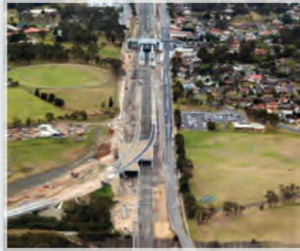
Glenfield Junction was a complex project that required innovation in design and construction to deliver a major junction upgrade, in a live rail environment with limited access. The careful use of innovative methods, segregation walls and precast concrete ensured efficient project delivery.
